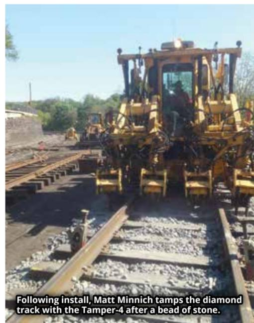
Following install, Matt Minnich tamps the diamond track with the Tamper-4 after a bead of stone.
