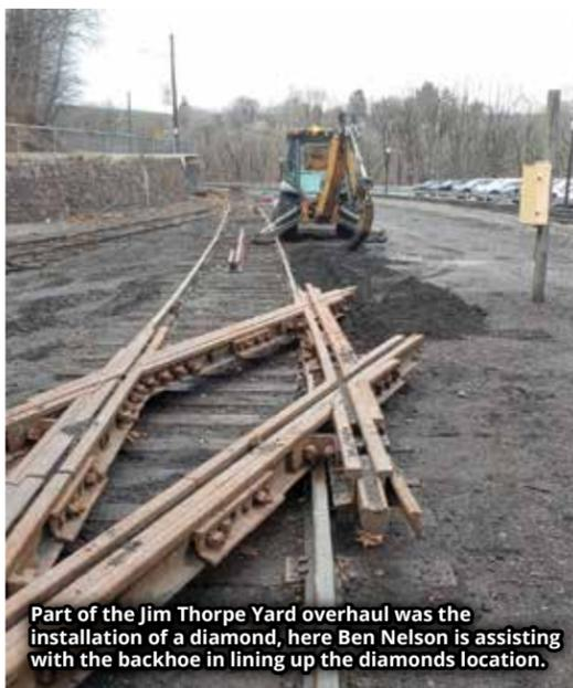
Part of the Jim Thorpe Yard overhaul was the installation of a diamond, here Ben Nelson is assisting with the backhoe in lining up the diamonds location.
