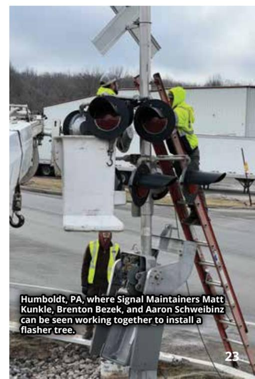
Humboldt, PA, where Signal Maintainers Matt Kunkle, Brenton Bezek, and Aaron Schweibinz can be seen working together to install a flasher tree.
