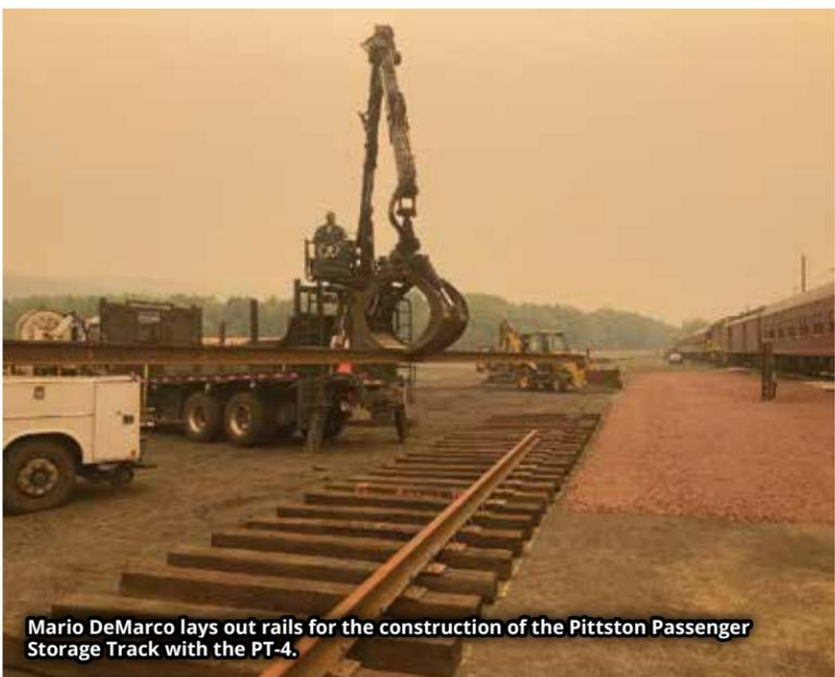
Mario DeMarco lays out rails for the construction of the Pittston Passenger Storage Track with the PT-4.
